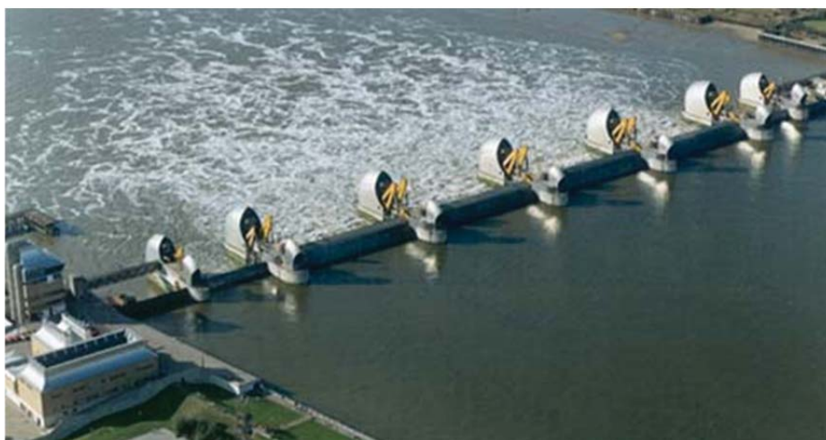
Figur 4.7: Thames Barrier i London
